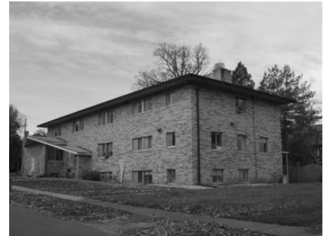
The Friendship House is located at 480 8th Street in Red Wing. The Statue of St. Thomas Aquinas is placed in the front yard. The beehive signifies a community of people caring for the needs of others which is a fitting symbol to the collaboration of non-profit organizations
